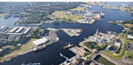
Access to key energy hub Wilhelmshaven, Germany
